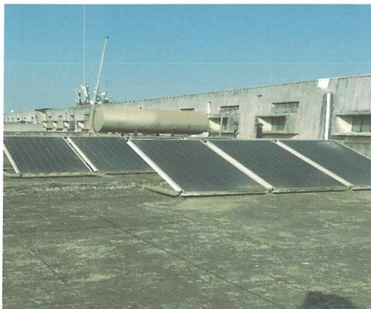
Photograph of Solar Thermal Water Heating Plant:
