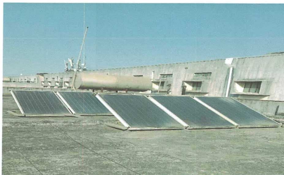
Photograph of Solar Thermal Water Heating Plant:
