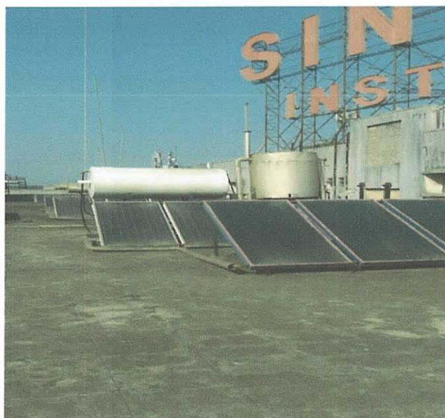
Photograph of Solar Thermal Water Heating Plant:
