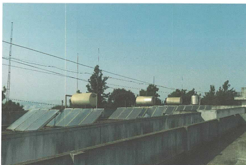
Photograph of Solar Thermal Water Heating Plant:
