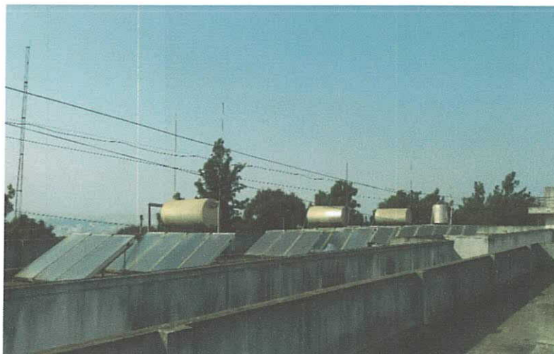
Photograph of Solar Thermal Water Heating Plant:
