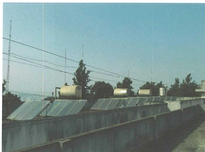
Photograph of Solar Thermal Water Heating Plant:
